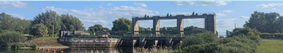
Figure 5. Sluice Gates at Denver
