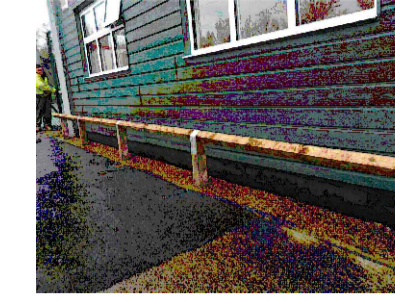
0.45m high timber knee rail fence (1:50)
