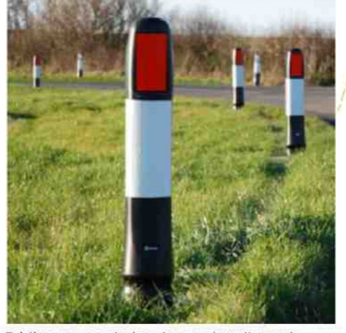
Existing access to be stopped up through installations of 600mm verge lined with Vergemaster Marker Posts and new access to be installed to county council standards
